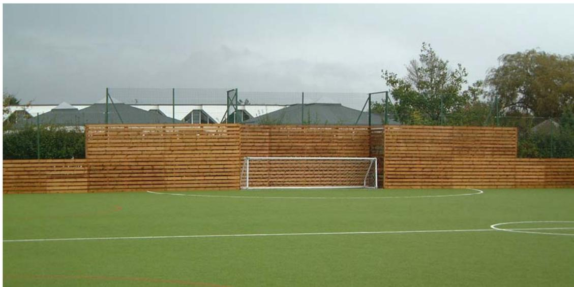
If timber planks or slats are used they should be smooth planed to a minimum thickness of 20mm. Mounting bolts for planks and panels should be roundhead on the inside face of the pitch. Suitable provision for expansion and contraction of the boards or planks should be allowed for in the design.
