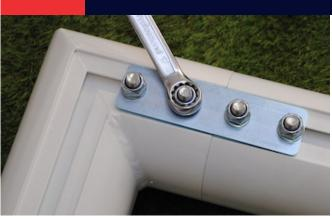
It's vital that you check bolts are tightened and securely fastened as loose nuts and bolts can cause a number of issues. The goal will become unstable, pieces will fall off during play, and there will be increased wear and tear on other parts. This is a simple fix as many goals use the same size parts, so a quick turn with a 17mm or 13mm spanner can eliminate many future problems.
