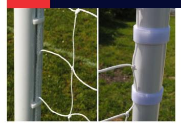
Replace any net hooks that are missing or broken. Nets that are not properly fastened to the goals not only look untidy but can cause a real safety issue with an increased chance of players becoming tangled in the net. If the goals are aluminium they will most likely use an enclosed hook that slots into the moulded channel of the goal. With steel and plastic goals that don't have this channel, Velcro or cable ties can be used to secure the nets to the posts.
