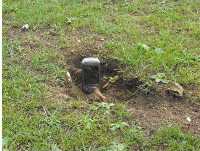
Figure 8 - Sunken drainage channel
