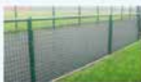
1) 1.2m in-filled pitch perimeter barrier to divide spectator area from FTP surface
