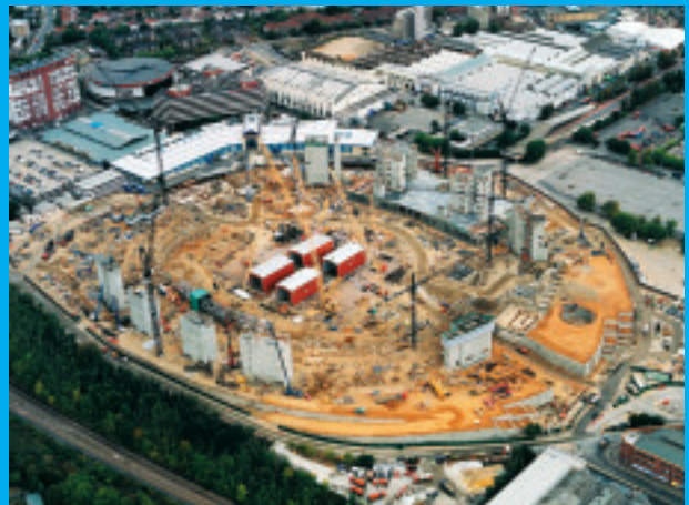
With foundation work complete, the new stadium is rapidly emerging
