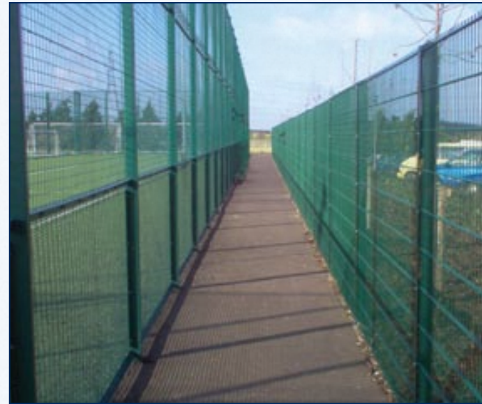
Secure access from changing rooms prevents pitch access contamination.
