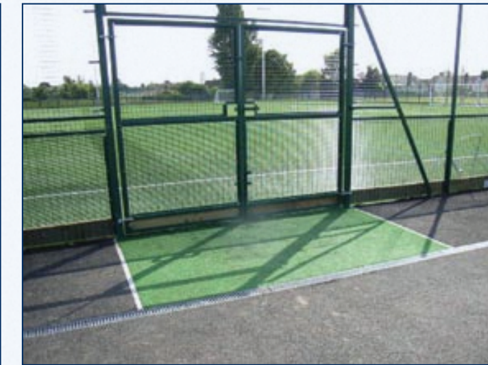
Use of matting at entrances to prevent contamination of pitch
