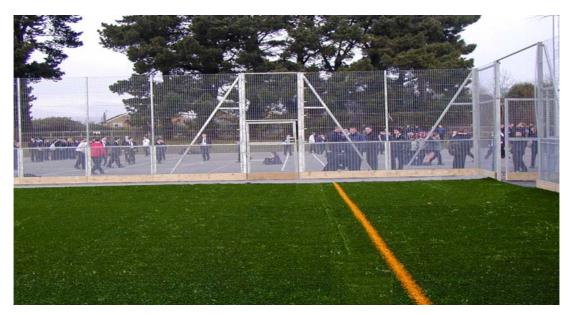
Access gates and doors should open outwards to ensure the safety of players. Single gates should be at least 1.2m wide to allow sport wheelchair access and gate thresholds should be level or slightly ramped (i.e. not stepped). Gates should also be positioned so they do not to create congested gathering points.
