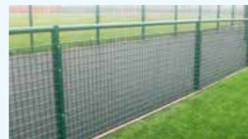
1) 1.2m in-filled pitch perimeter barrier to divide spectator area from FTP surface
