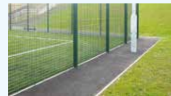
6) A minimum 300mm mowing strip around outside of fencing to protect bounding boards and fence
