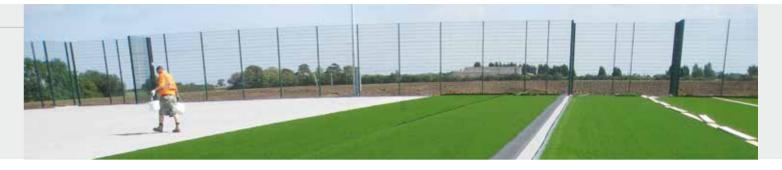
The largest pitch markings on the 3G FTP should always be white and training lines should always be red. These lines should be tufted in during the manufacturing process. The rest of the lines should be marked on by following these principles:
